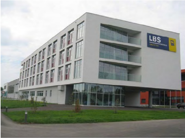
Fig 12: Vocational school in Amstetten, Austria
