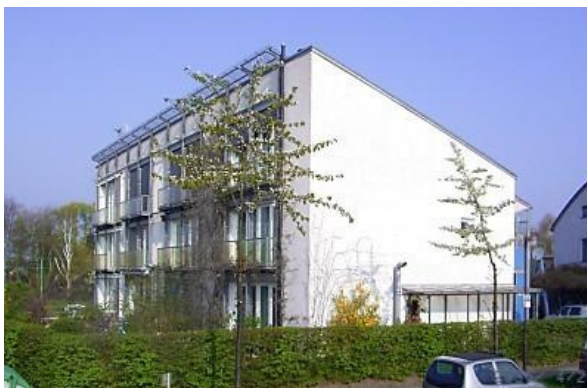
Fig7:Passive House Darmstadt Kranichstein
