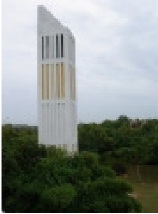
Air Conditioning Tower Images from:
