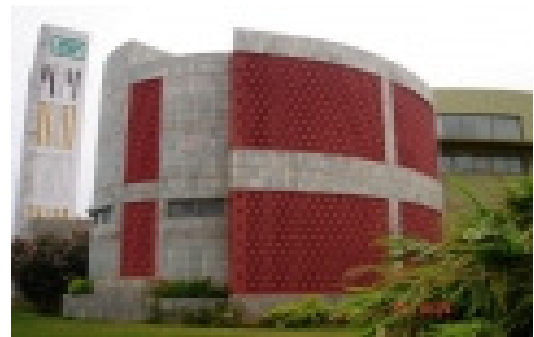
Recycling Materials construction
