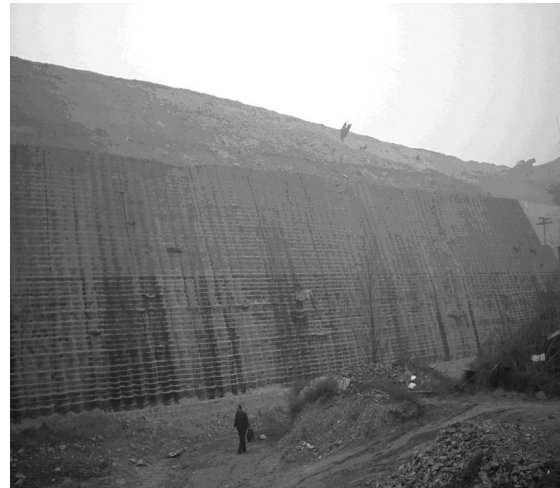
Figure. 5 Geocell flexible retaining walls.
