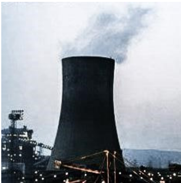
Fig 3 (a) Sipat Thermal Power Plant
