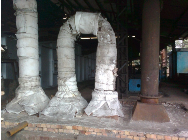
Fig. 4: Insulation of pipeline of recuperator
