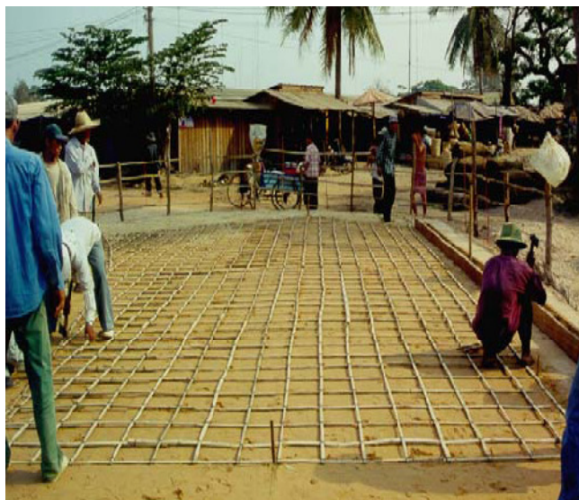
Fig. 1 Preparation of bamboo reinforcement
