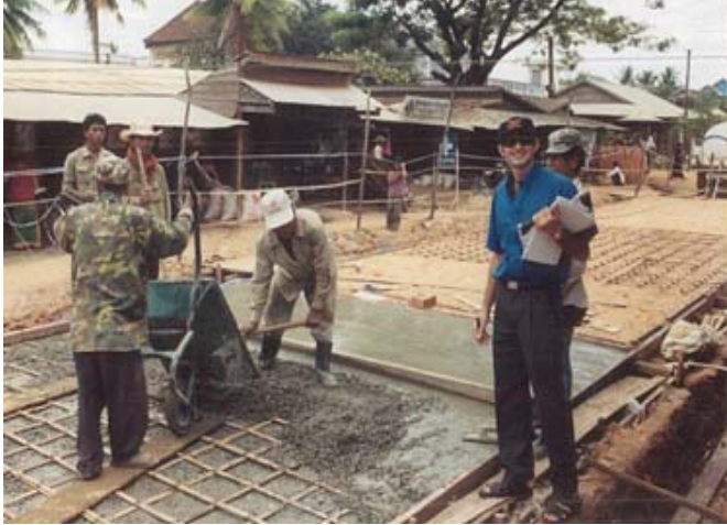
Fig. 2 Placement of concrete and compaction
