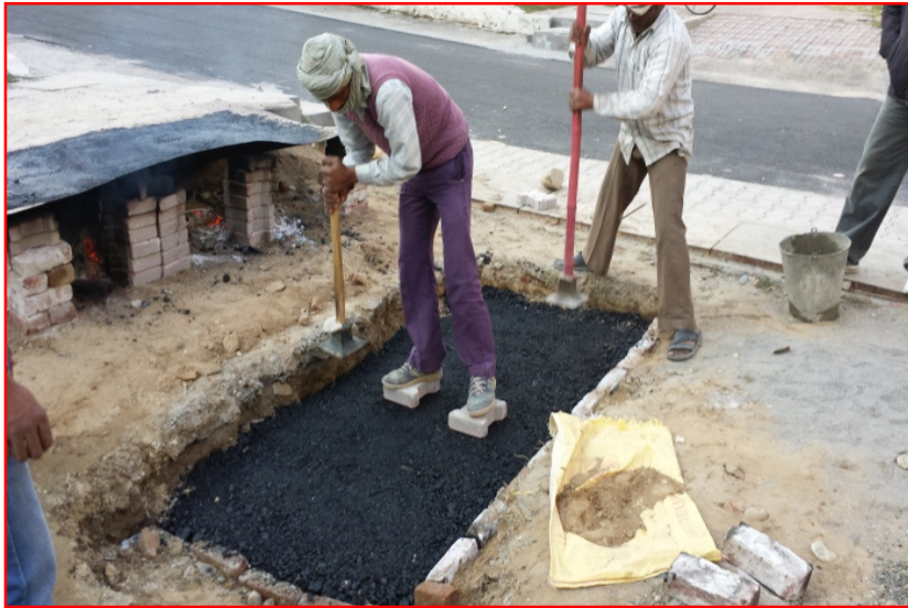
Fig 4 Construction of Test Track for FWD Testing
