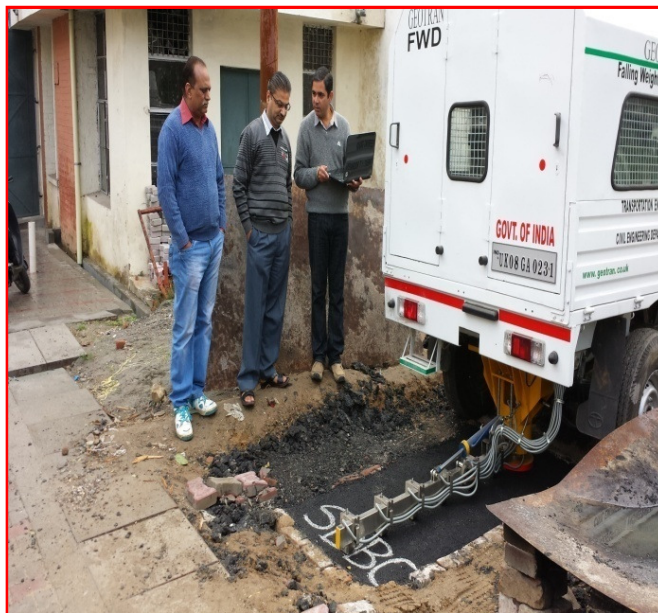
Fig 5 FWD Testing of Test Pavements & Other Chosen Locations
