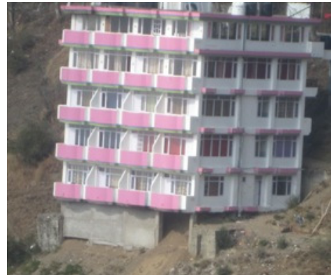
Fig. 12: Construction of Shear wall
