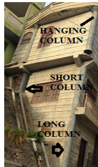
Fig. 6: Floating and short columns
