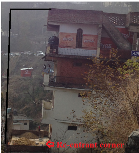
Fig. 7: Setbacks (Re-entrant corner)
