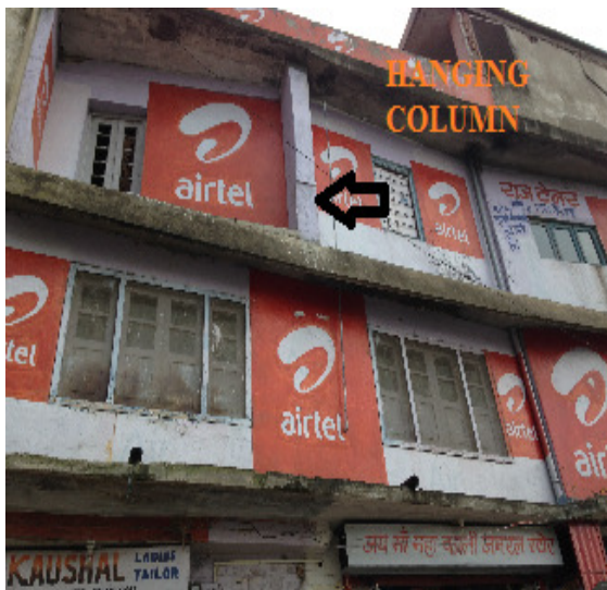
Fig. 5: Hanging columns or Floating columns
