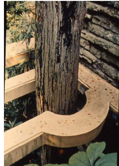
Figure 7 Tree was not cut but the design of trellis near the front door was changed to semi-circle
