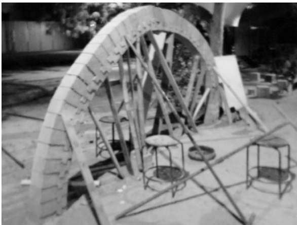
Figure 1 :papercrete interlocking arch made by jil,dhruv,shivam,aakansha and devisha as a group.
