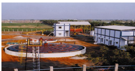
Fig 2 : 0.15 MW Power Project Utilizing Vegetable Market and Slaughterhouse Wastes at Vijayawada, A.P.
