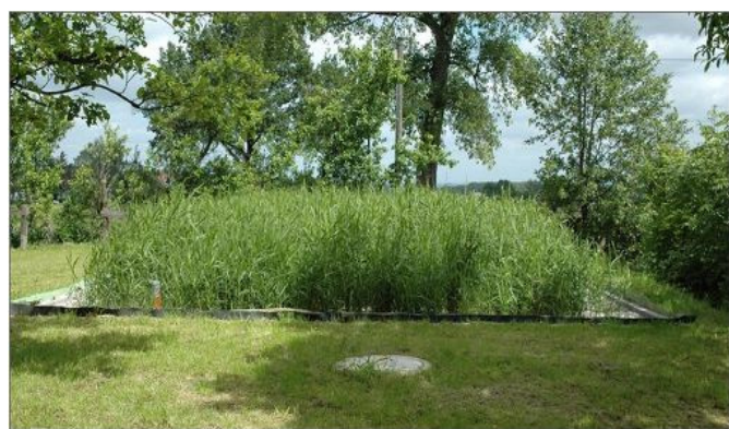
Fig. 2. A diagrammatic and actual field picture of a sub-surface constructed wetland
