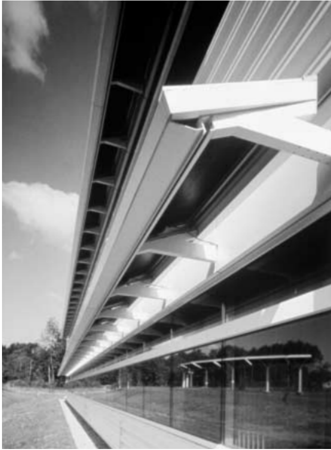
Fig. 2: PV as A Shading Device [2]
