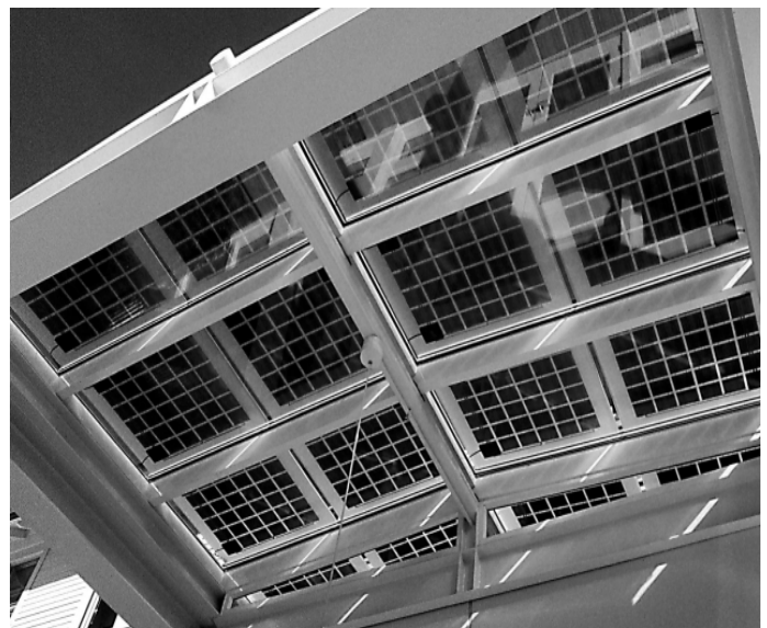
Fig. 1: PV as skylight [1]
