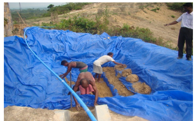
Fig. 3. Stepwise construction and lining of RHS.
