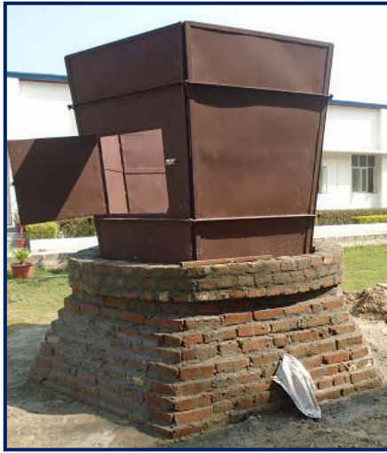
Fig. 2: Actual acoustic shield installation in progress
