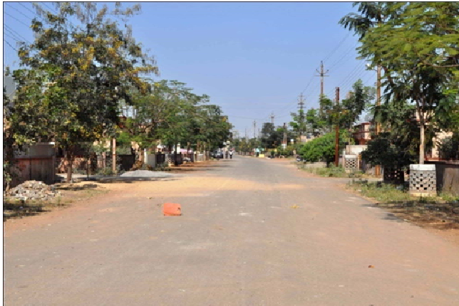
Fig. 9: 19 metre wide internal road
