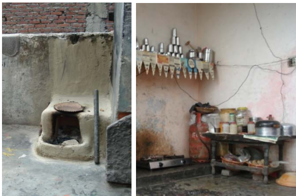
Fig. 8: Semi open Kitchen on First Floor
