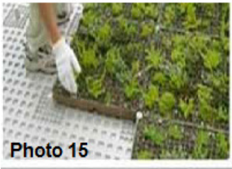
Photo 15 4. Install Modules
