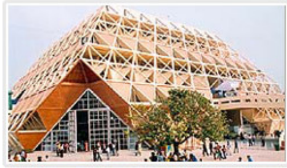
“Fig .3.1” exterior view of Hall of Nation
