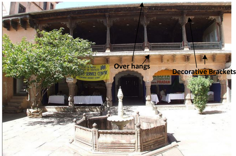
Fig6: The shading device supported with decorative stone brackets. Source: www.flickrriver.com
