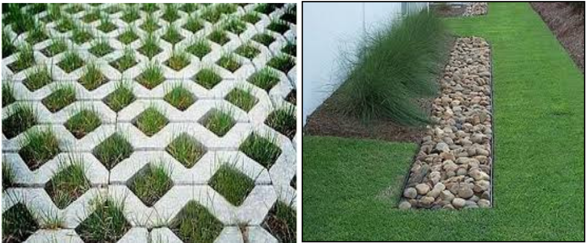
Image7: Porous pavement for pathway. Source: http://www.lastormwater.org/green-la/low-impact-development/residential-solutions/permeable-pavements-or-porous-pavement-systems/
