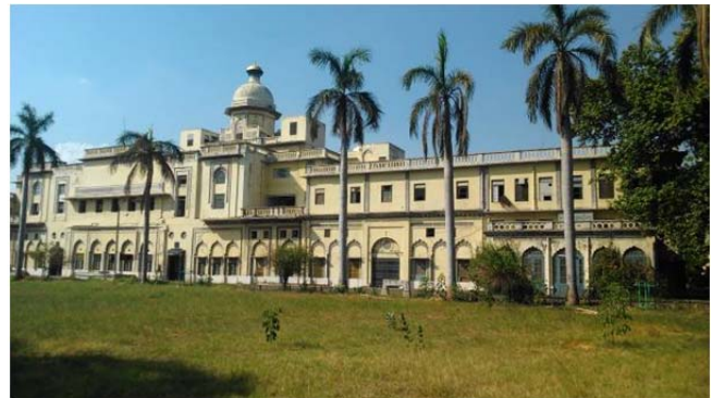
Fig. 2: Front view of the Chattar Manzil Kothi
