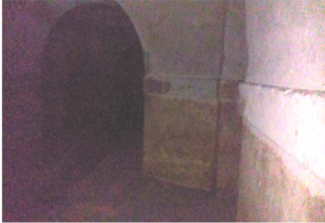
Fig. 10: Basement with semicircular arch
